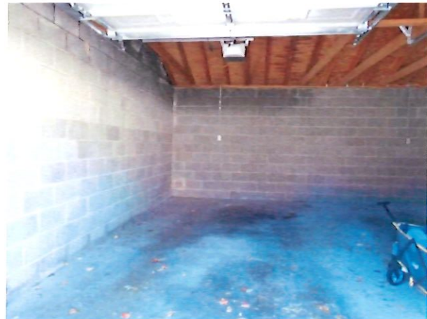
Interior typical Garage
