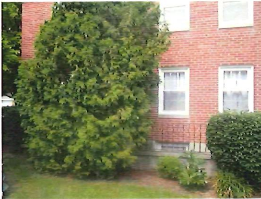
Additional Front View of Lower Level Windows
