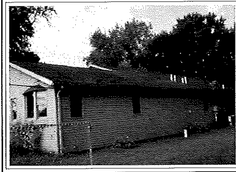
View of north side
