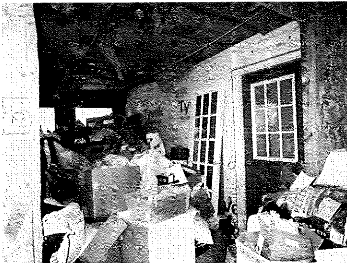
Rear Enclosed Porch
