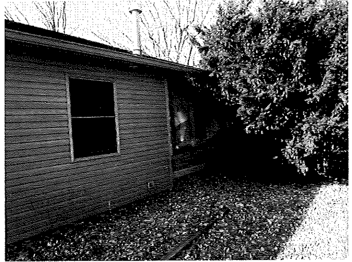
Additional Exterior View
