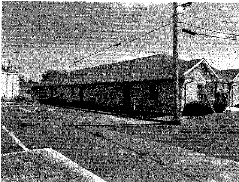
Extra Photo for Back of Building: West side of the building
