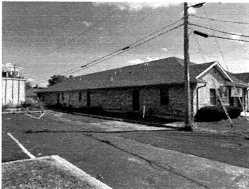
Back of the building: West side of the building
