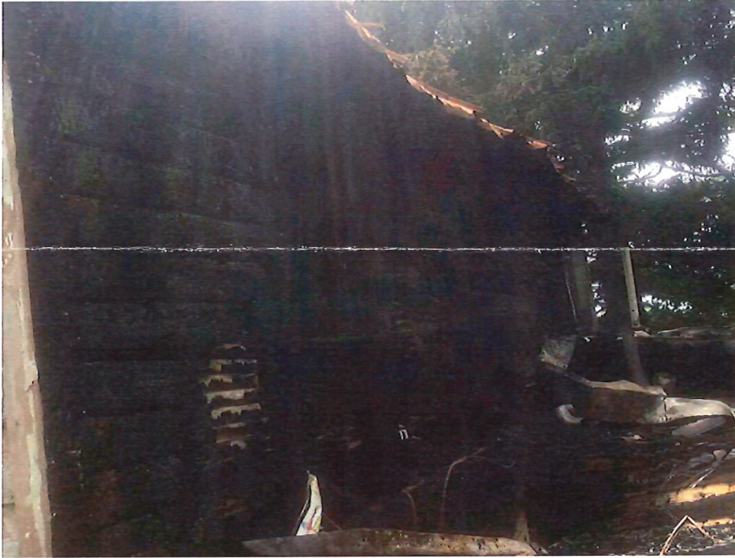
11-Rear elevation, fired damaged siding.
