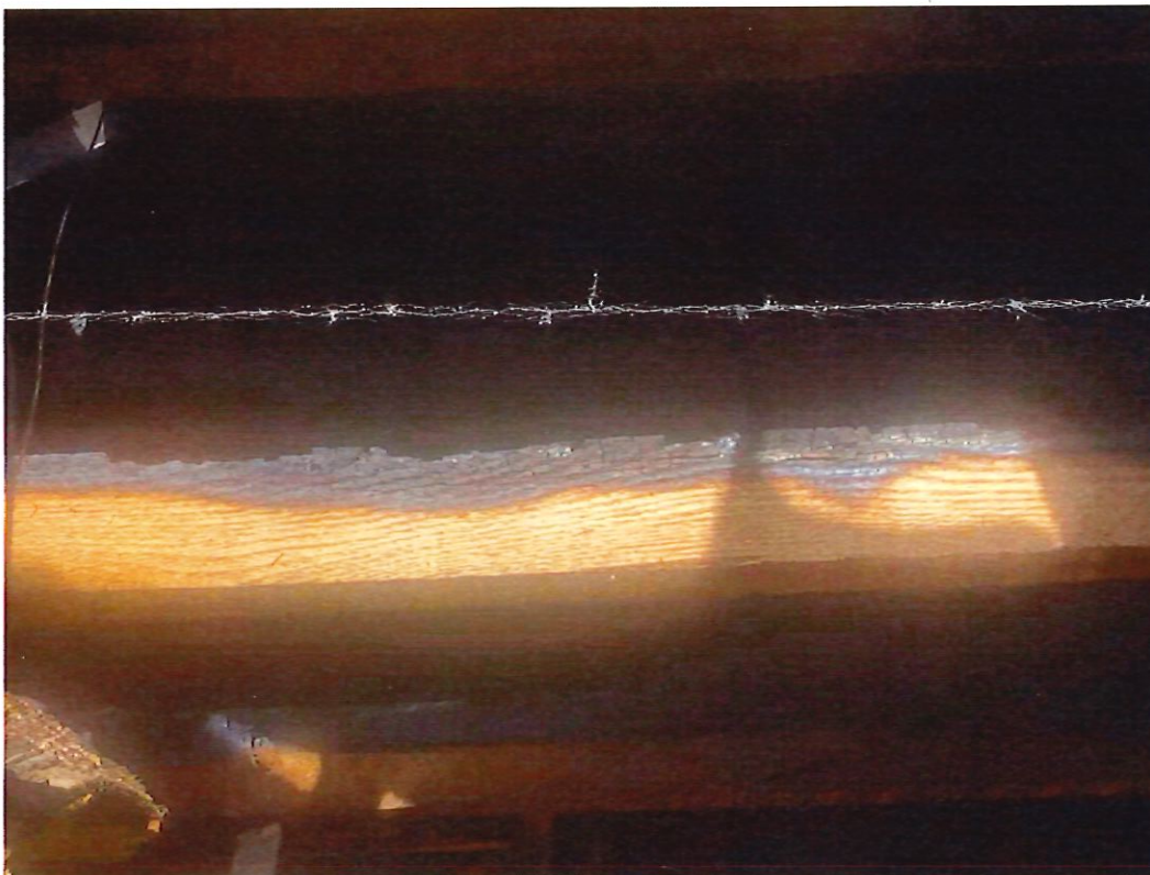
26-Bedroom, fire damaged trusses and sheathing.
