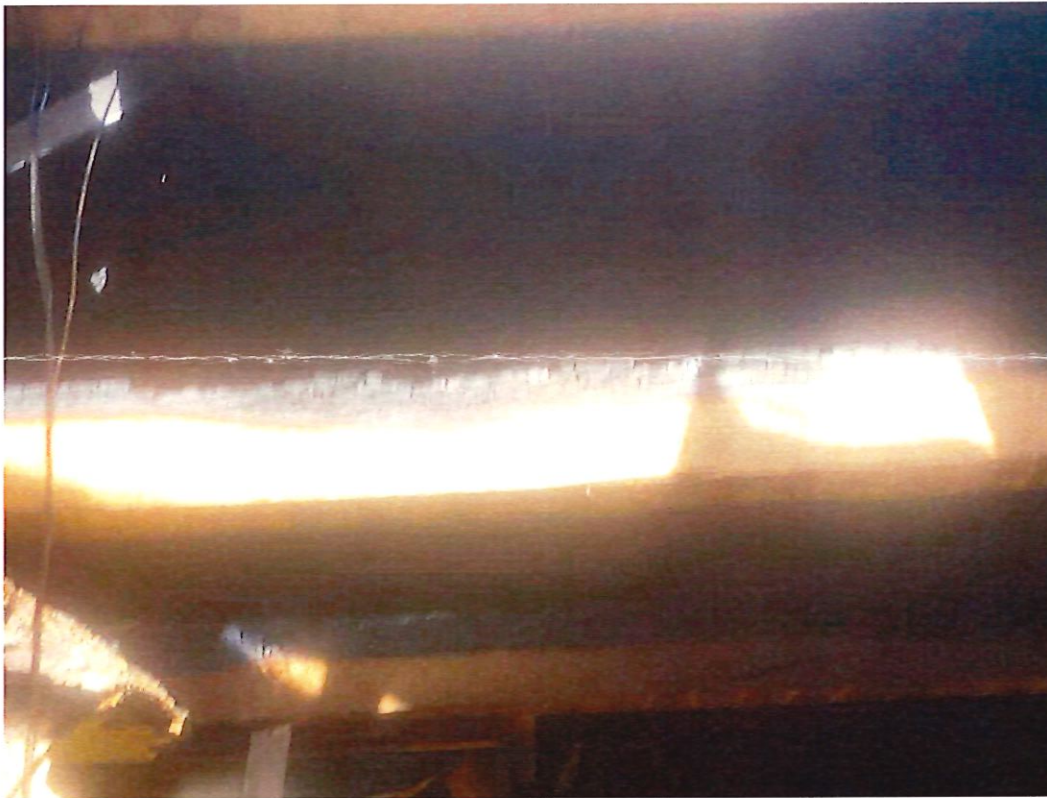
25-Bedroom, fire damaged trusses and sheathing.
