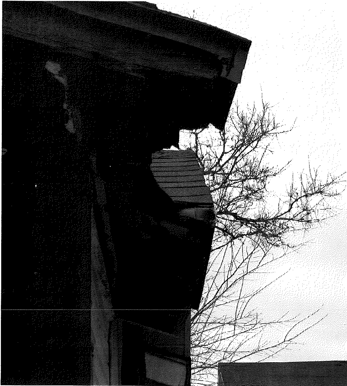
Roof damage sustained from neighbor's tree falling on house.
