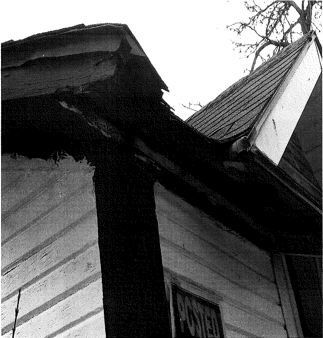
Additional picture of roof damager.
