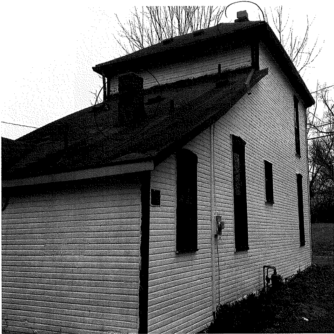
View showing patched roof and both Chimneys.
