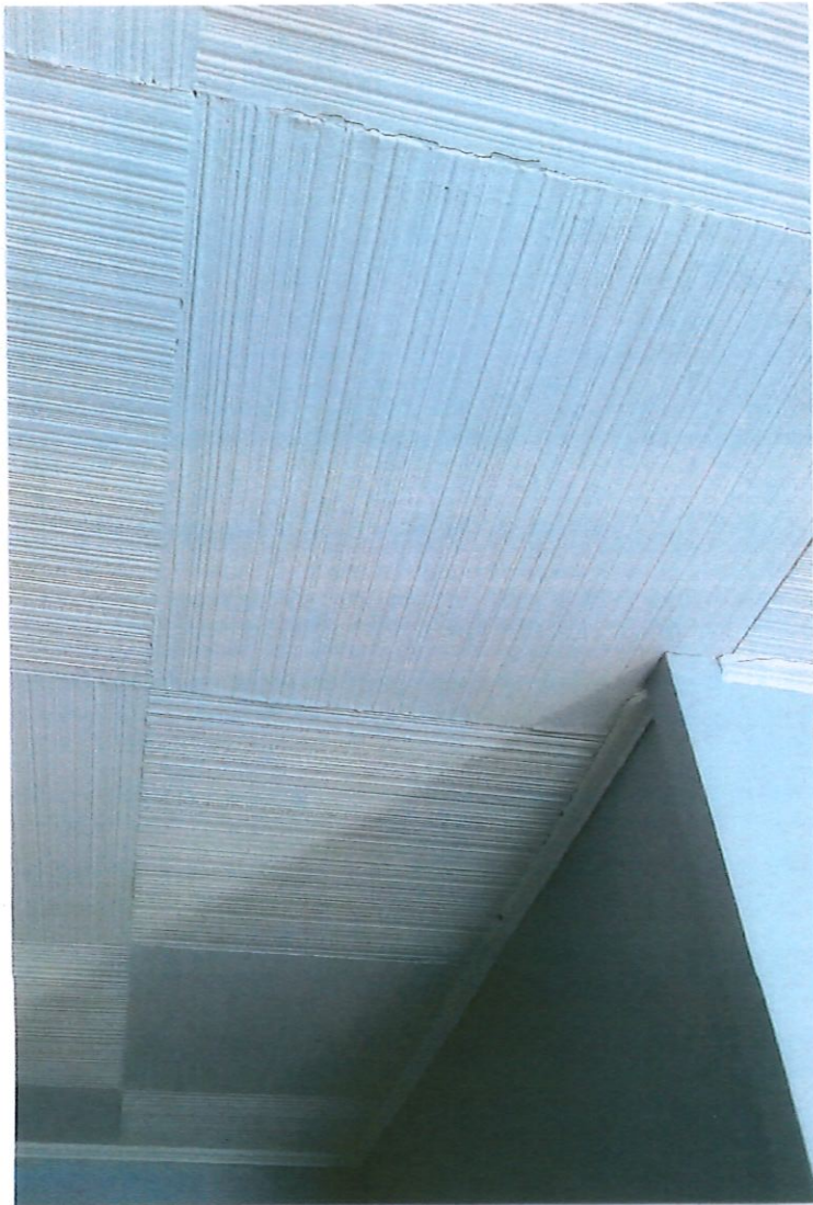
LIVING ROOM CEILING (OLD STYLE)
